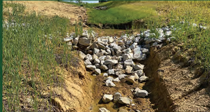
Fully vegetated InstaTurf vs Rock Riprap in Channel
